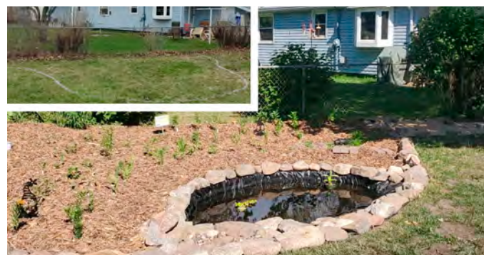
Before and after: Installation of a 250 sq. ft. residential raingarden
