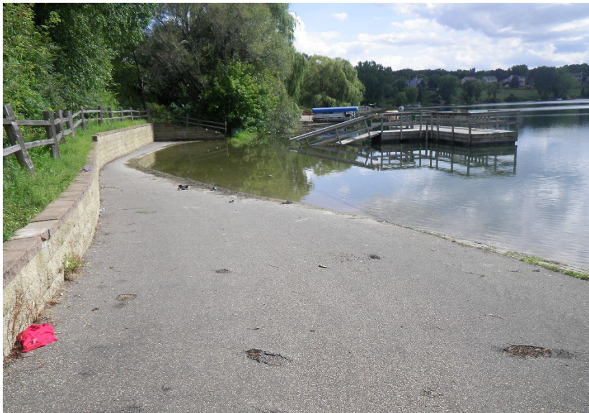
Photograph 2: High lake levels in 2019 preventing access to the Lac Lavon fishing dock in city park.
