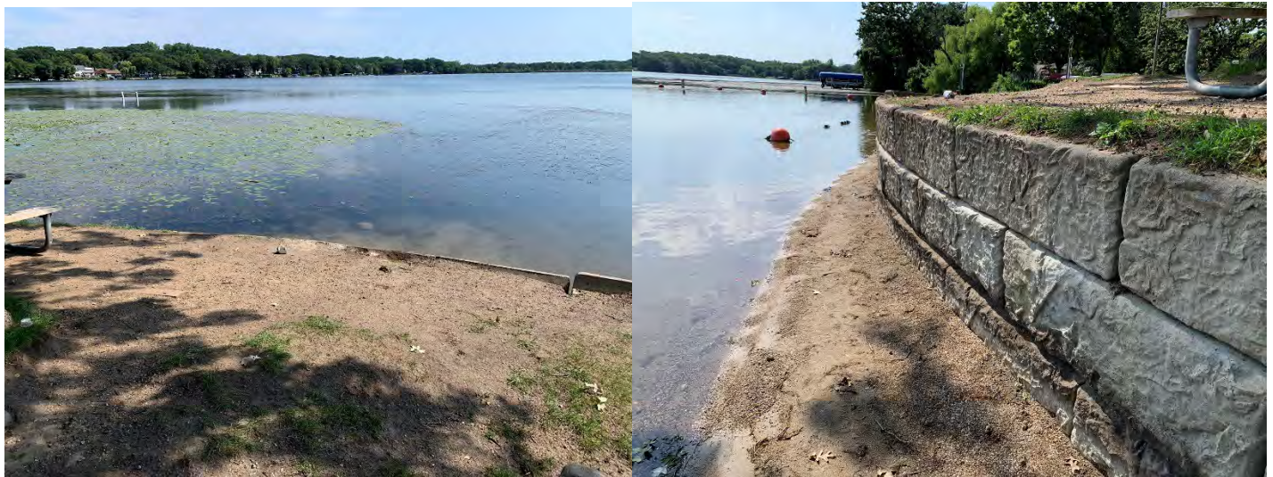
Timber wall was replaced by concrete wall at north end of beach area. Poor vegetation establishment and trash above the concrete.
