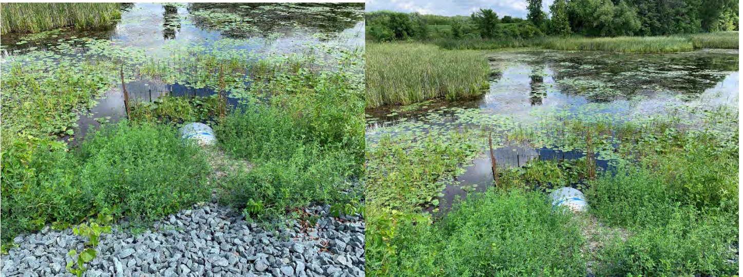
A new culvert under railroad tracks was installed under railroad tracks to maintain flow through of surface hydrology between Areas B and C.
